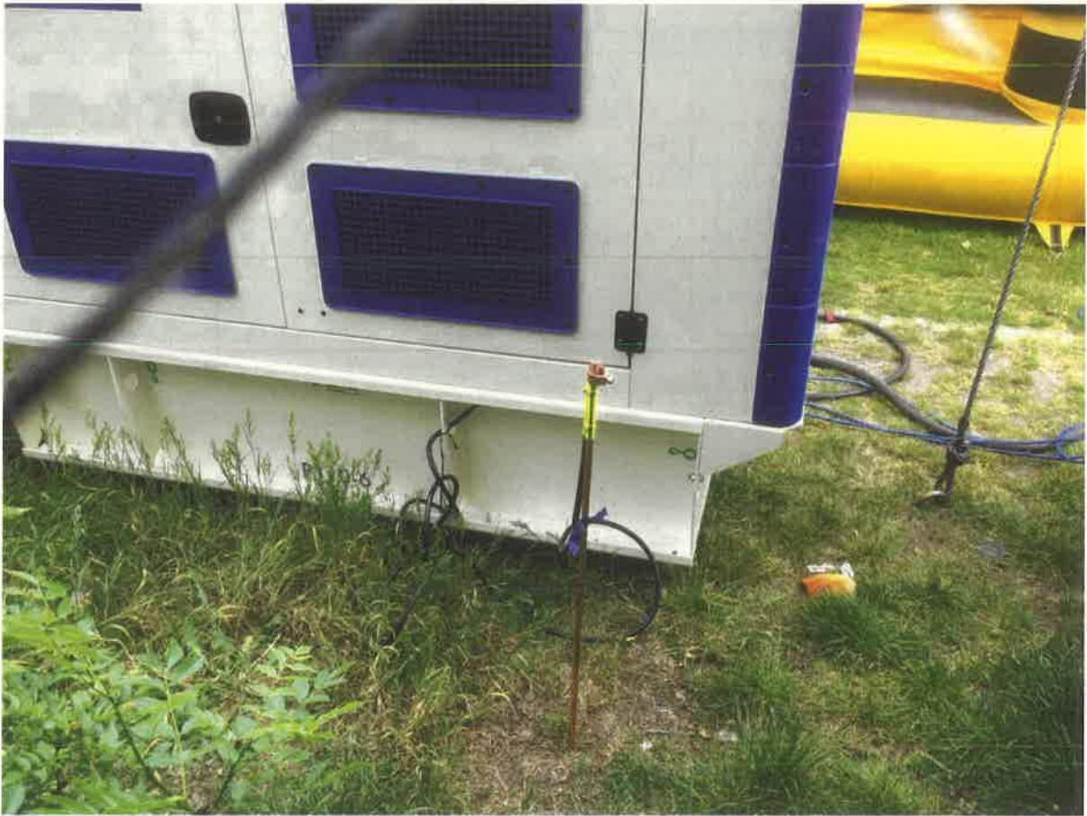
Insufficient Earth to Generator
